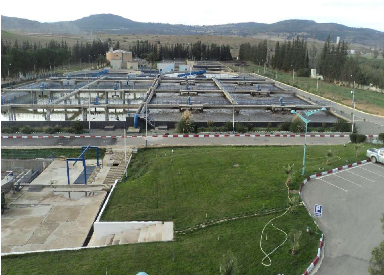
Figure 19: Overview of the treatment plant of the province of Saida
